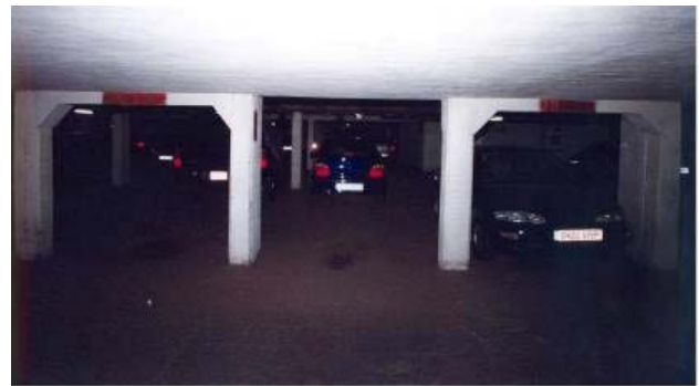
Figure 11. Portico pillars in the parking lot.
