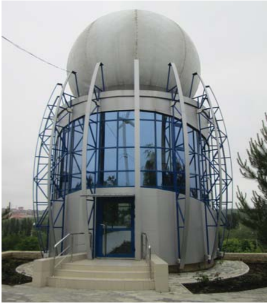
Figure 2. Ground station with parabolic antenna, 9 Studentilor str., Chisinau
