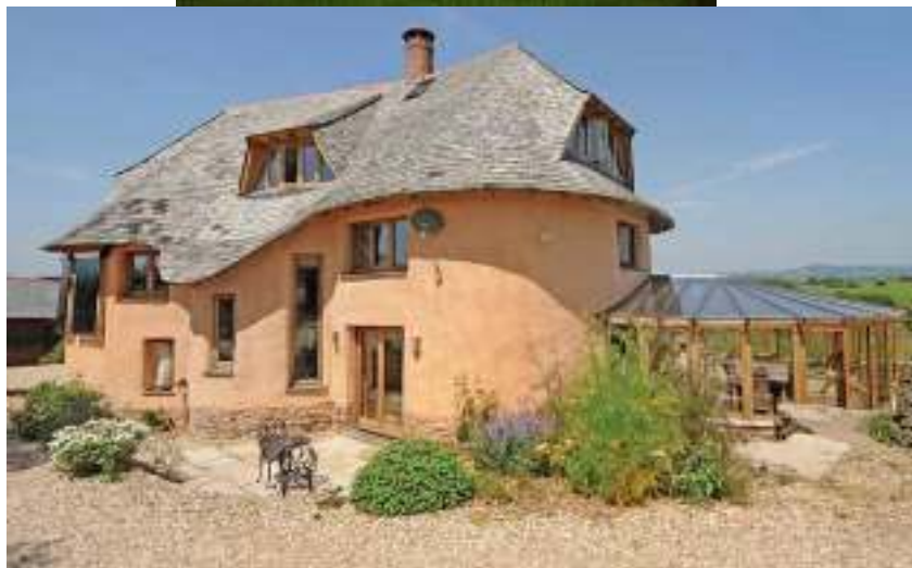
Fig. 1. New clay houses constructed cob building specialist Kevin McCabe 1 mile from Ottery St Mary town centre unique design of houses built of clay, based on the concepts of organic architecture.
