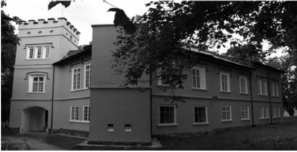
Figure 2. Country Palace de Zotte, Vykno village, Zastavnovsky district (photo by A. Bondarenko) [12]
