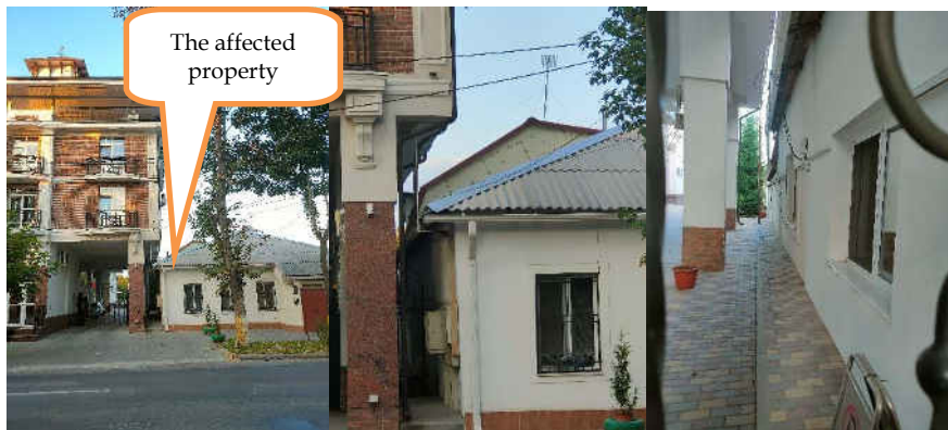
Fig. 4. Full room shading. Source: original photo taken by the authors.
