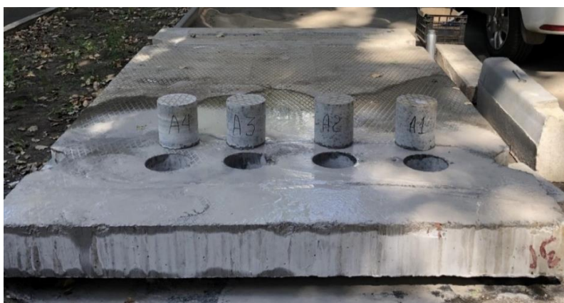
Figure 7. Drilled cores of the slab
