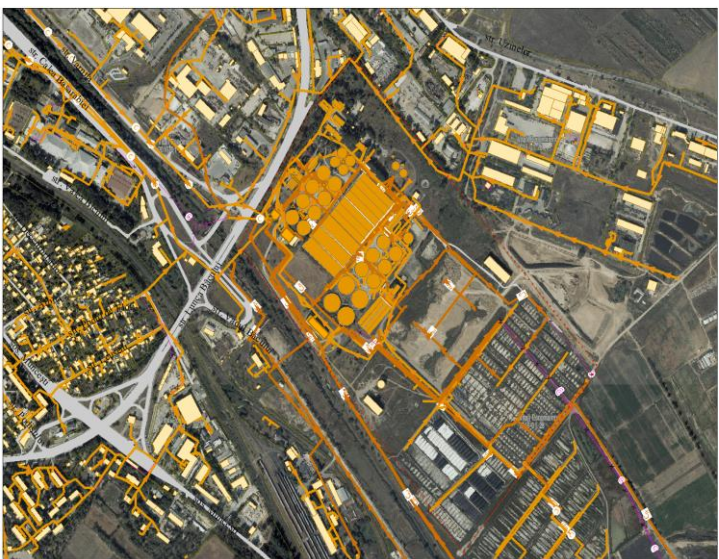
Fig. 1. The Chisinau wastewater treatment plant.
