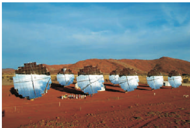
Fig. 2.93. Concentrator paraboloidal PV: Sistem Solar Pty, LTD (Sursa: NREL).
