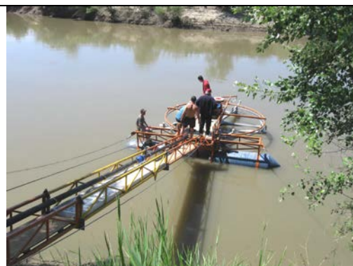
Figure 8: Testing of the industrial prototype of micro-hydro power plant on the Prut river.
